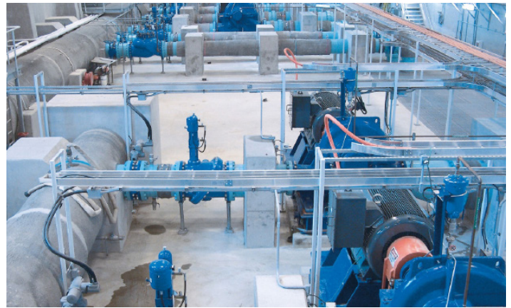
Beckett Sproule Pumping Station
